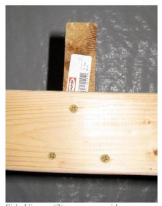
Side View – (3) screws per side, (2) two in the 2"x4" and (1) one in the 2"x6"
